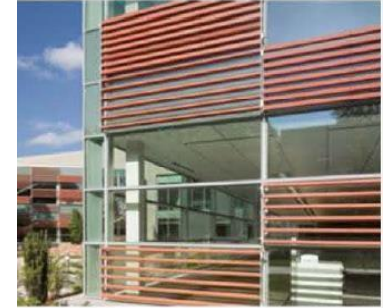
Double skinned Façade design to reduce heat ingress
